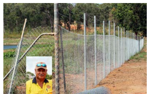
Sewer Ponds Fencing
