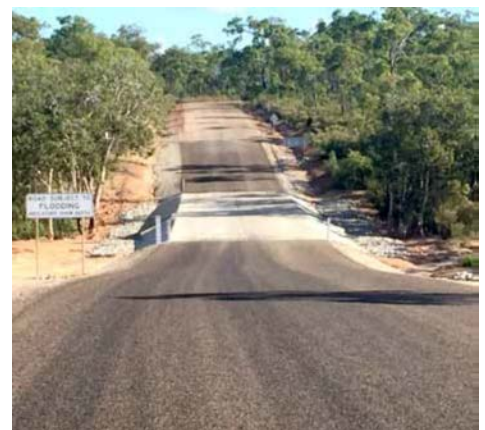
Sealed Road Works
