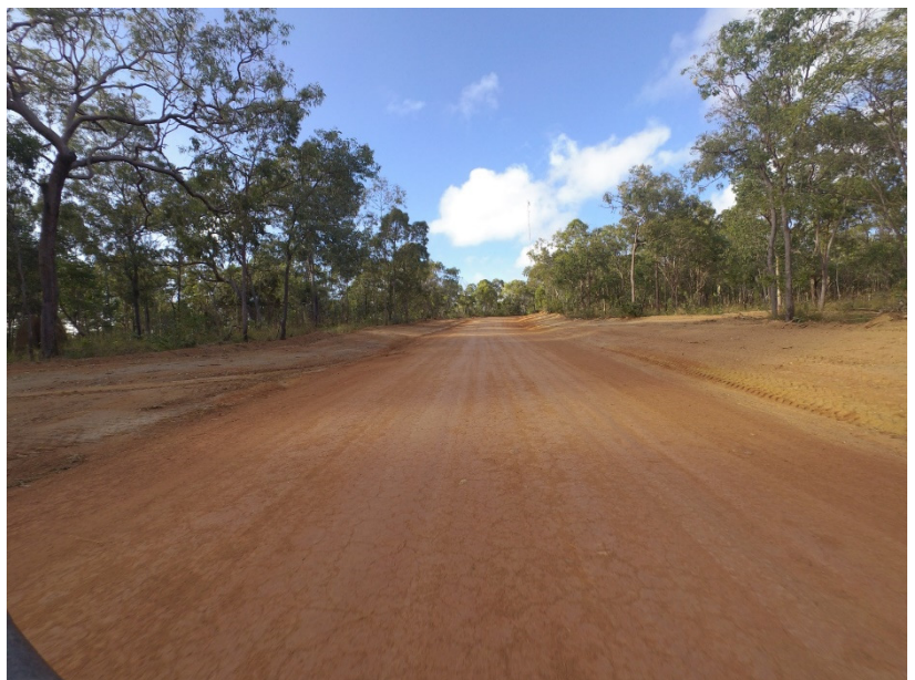
East Kuttini Street road works
