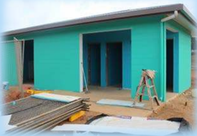
Water Park construction
