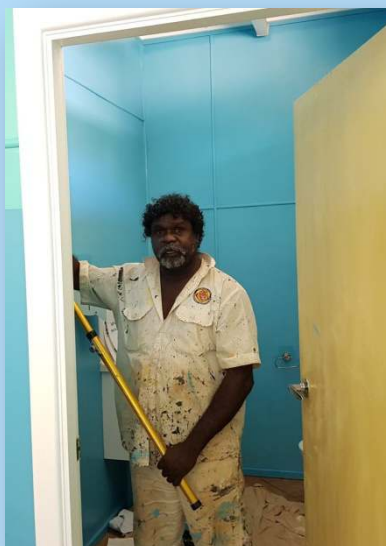
James Macumboy Carrying out Internal paint works
