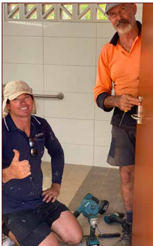
Rod working with a contractor at the new camping ground facilities.
